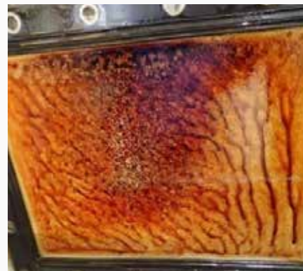
RESERVOIR HATCH COVER
